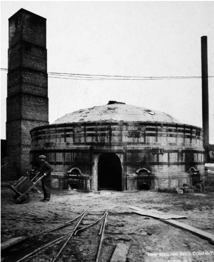
( m. ) New England Brick Company kiln, next to the clay pit which is now Danehy Park.
